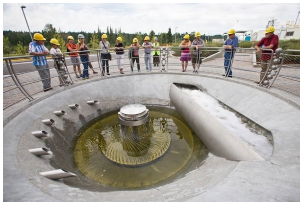
Jann Rosen-Queralt, "Confluence" detail, 2011. Photo courtesy of King County | Ned Ahrens (Brightwater Treatment Plant in Woodinville, WA)
